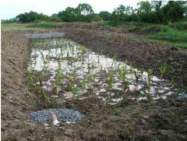
Newly planted wetland system for single dwelling, filled with clean water for planting and plant establishment.
