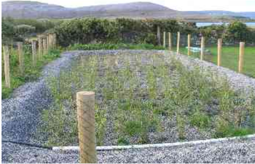
Newly planted reed bed system
