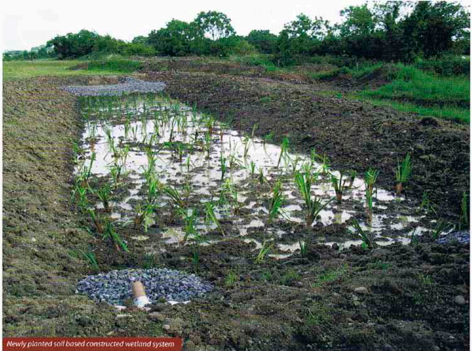
Newly planted soil based constructed wetland system
